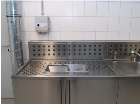
Disposal station with sieve insert and air draft system (downwards and backwards)
