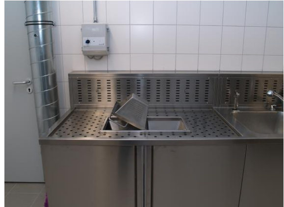
Sieve insert for separating liquids from solids
