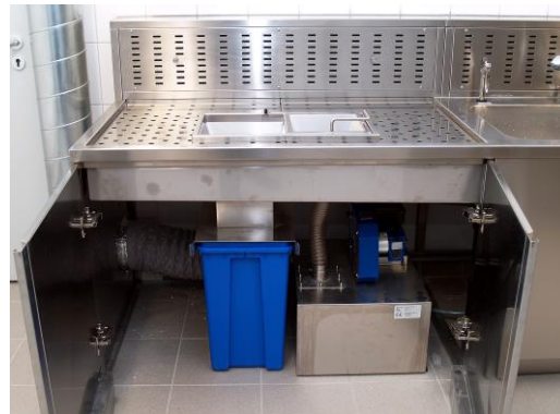
Disposer for solids / 60 litres container with formalin pump with automatic pumping system (customized solution)
